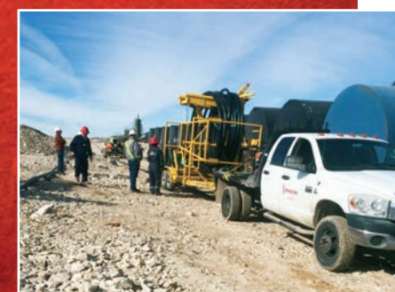
Flow Line Installation
