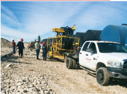
Flow Line Installation
