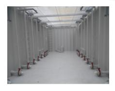
Each long side fitted with 6 - 8" flanged nozzles with internal valves, and 12 - 4" female threaded pipe couplings with internal valves. All fittings near floor level.
